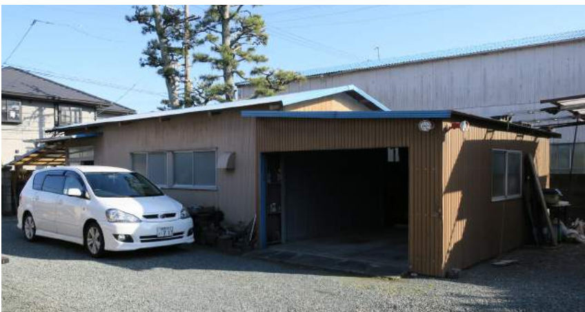
Middle left; This building is his show room filled with hundreds of different types of stones for sale.
